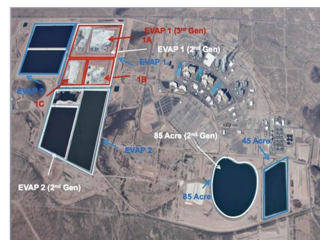
Figure 2: Evaporative ponds at Palo Verde
